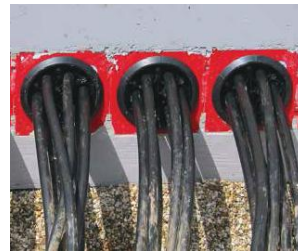
MULTI CABLES-PIPES TRANSIT SEALING SYSTEMS
